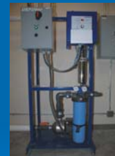
Photo 3: Filter Cartridge and UV Light
